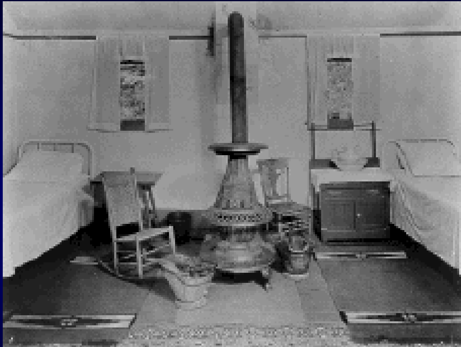
Interior view of "Little Red" New York 1884
